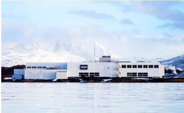
Insula headquarters and production facility in Leknes, Lofoten
